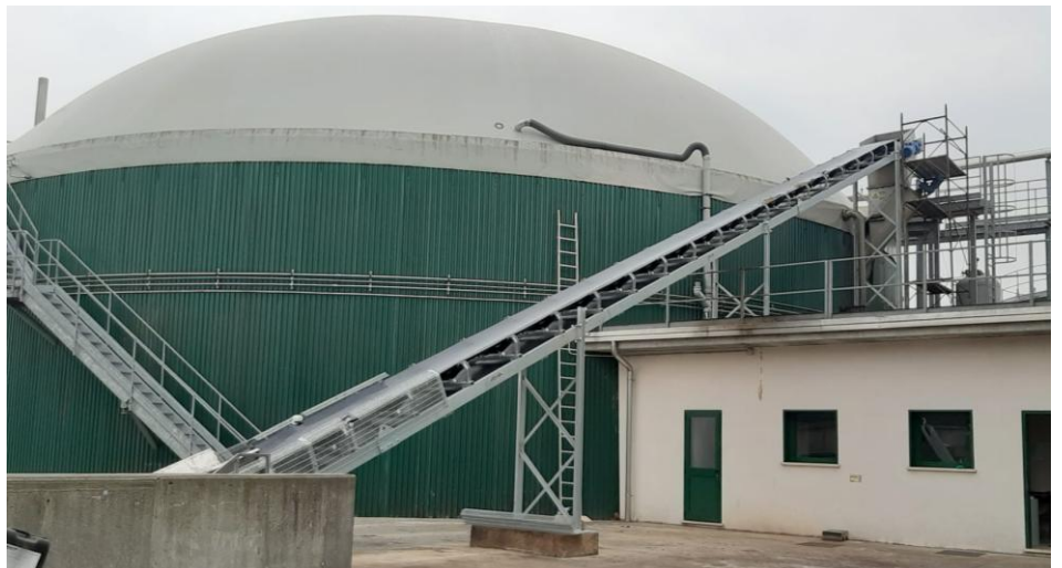
Customized TNV with rubber belts for raw materials feeding in Biogas / Biomethane plants
